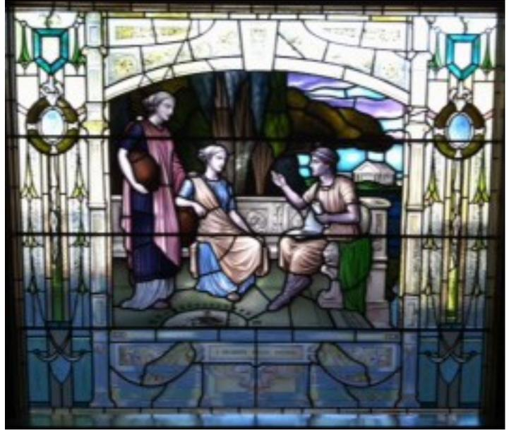
Laura and John photographed the window then made a rubbing of it to act as a guide for putting the window back together. Next, came the removal! Luckily, a flat roof is just below the window, so after protecting it with foam and plywood on the inside and out, the window was lowered onto the flat roof then large portions of the lead were cut and the window was divided into sections. These sections were then packed and John took them back to his shop.
